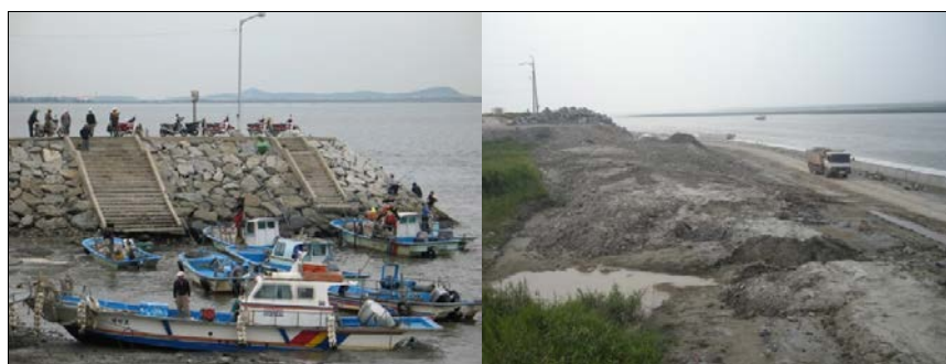
Fig. 2. Simpo fishing port (2007) under construction for a yacht harbor (2014)
